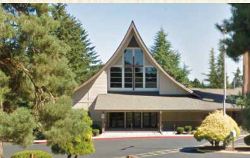
PHOTO: GOOGLE STREET VIEW
